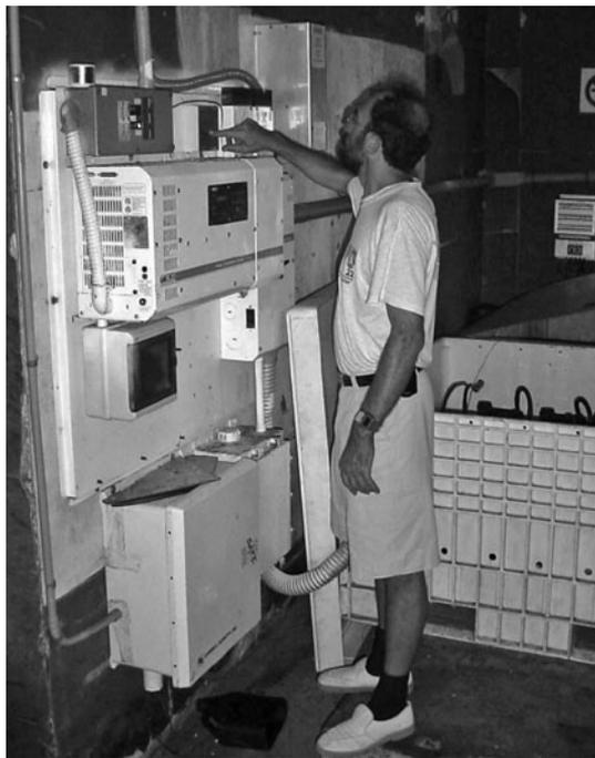
**FIGURE 8.25** Isla Contoy solar and wind energy power center, inverter, controls, and batteries.
