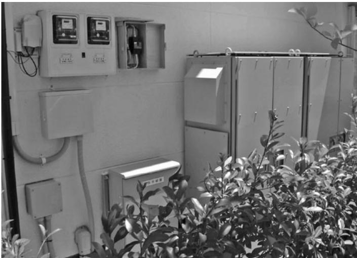
**FIGURE 8.6** PV system grid inter-tie (note 2 meters) in Ohta City. Inverter and battery bank are housed in the large boxes on the right.
