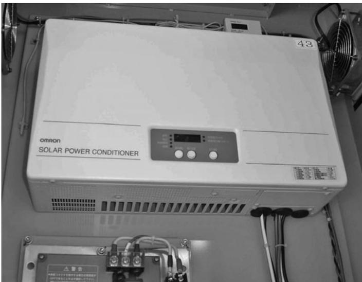
**FIGURE 8.9** Four-kiloWatt transformerless Omron inverter on AIST PV parking structure.
