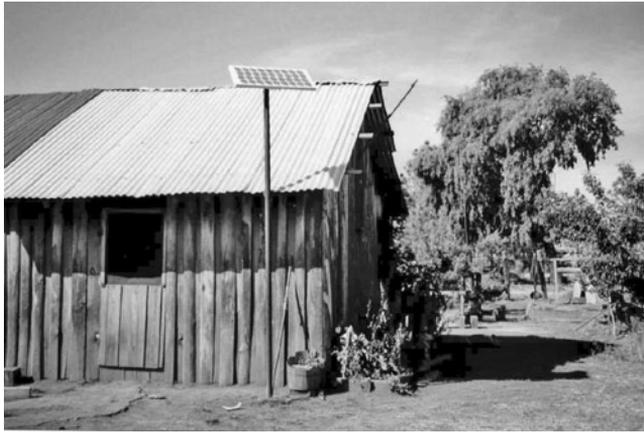
**FIGURE 8.17** Solisto 50 W<sub>p</sub> PV lighting system installed in Talayotes, Moris County, Chihuahua.
