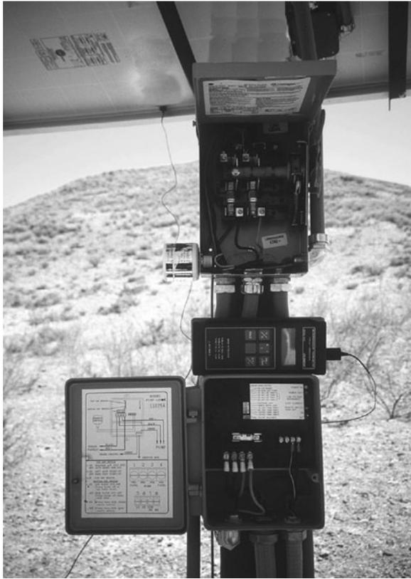
**FIGURE 8.39** Typical pump controller with overcurrent protection for PV water-pumping system in Chihuahua, Mexico.
