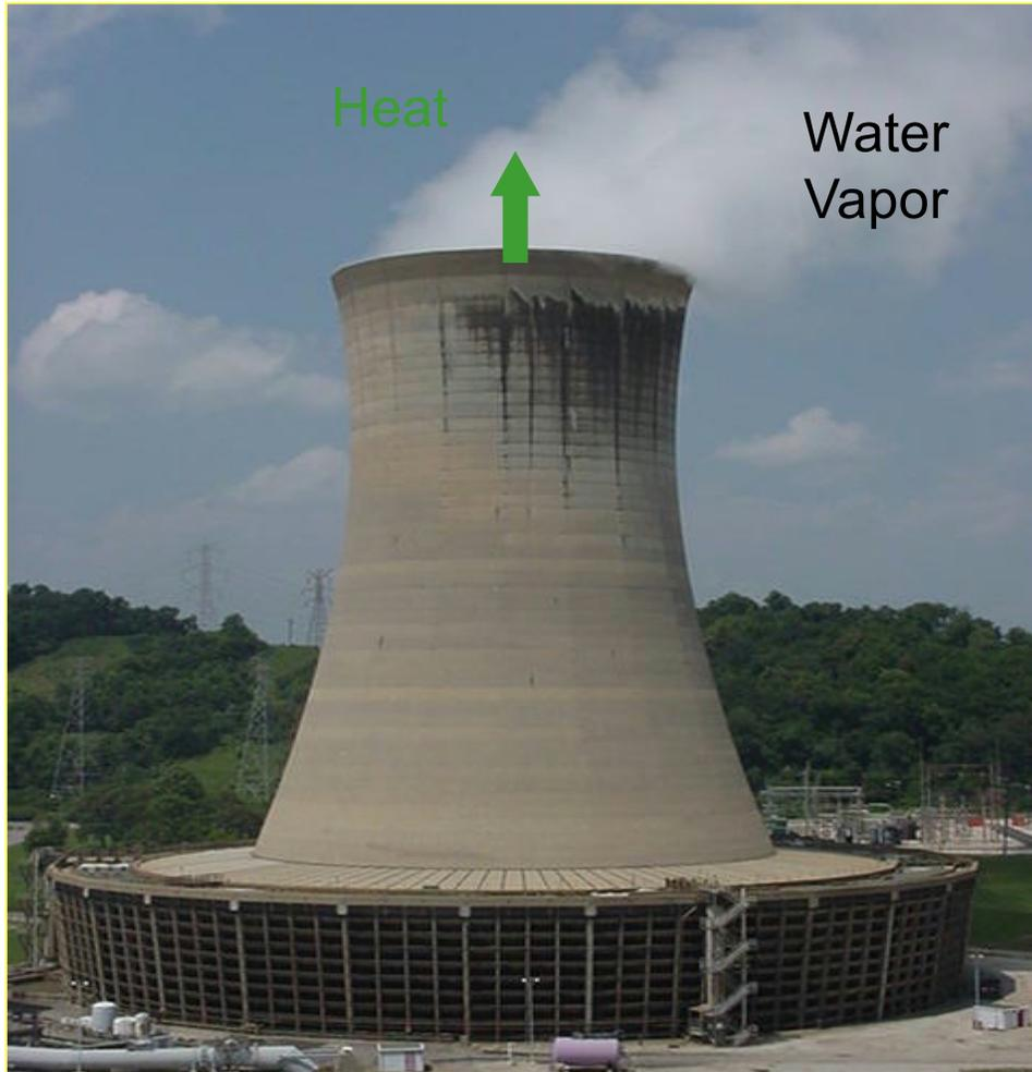
The circulating cooling water is cycled between these types of towers and the condenser. The heat in the falling water is carried away by the upward air draft in the towers.
