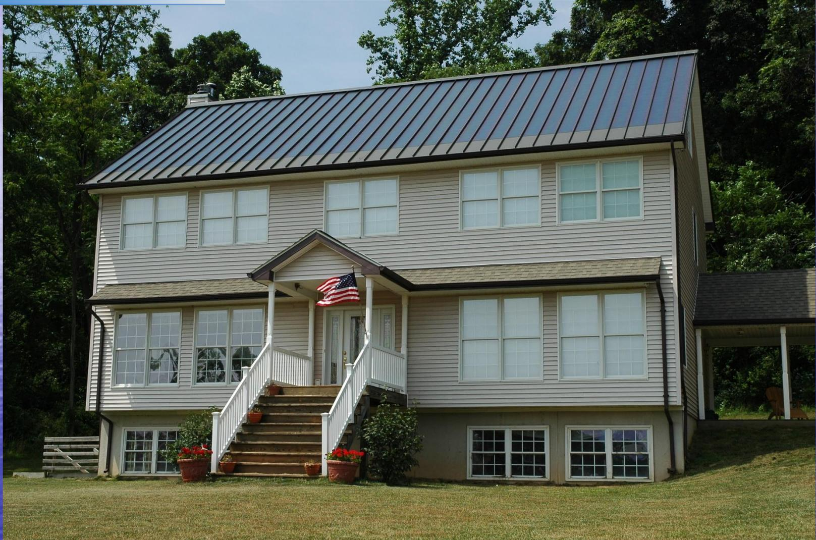
The Solar Roof features 36 PVL 128 Laminates from Uni-Solar . 4.0 kW
