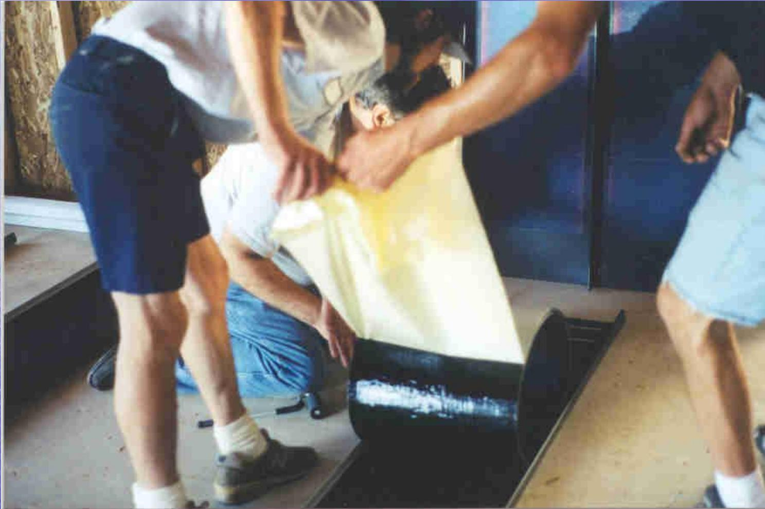
**The Uni-Solar PVL is applied to the Standing Seam Pan on site by the roofing contractor.**
