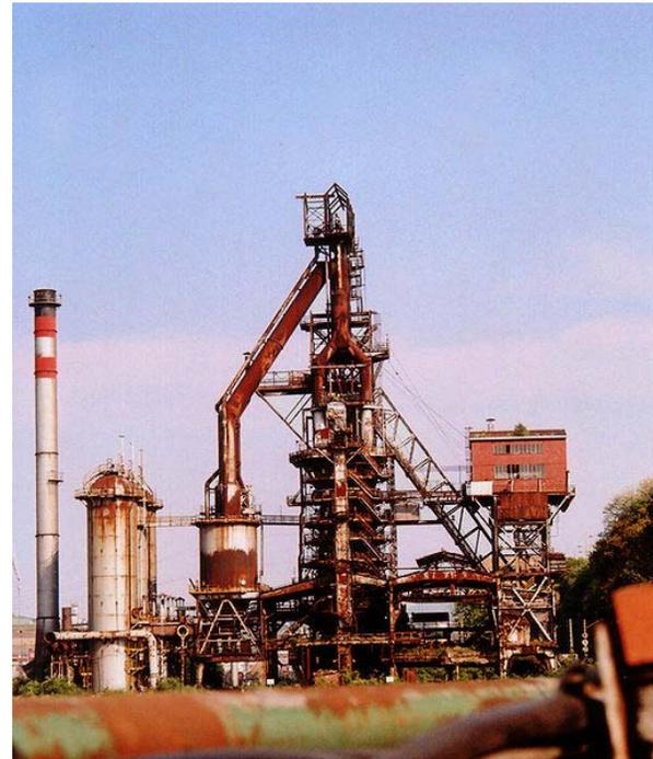
A **blast furnace** is a type of **metallurgical furnace** used for **smelting** to produce industrial metals, generally **iron**.
