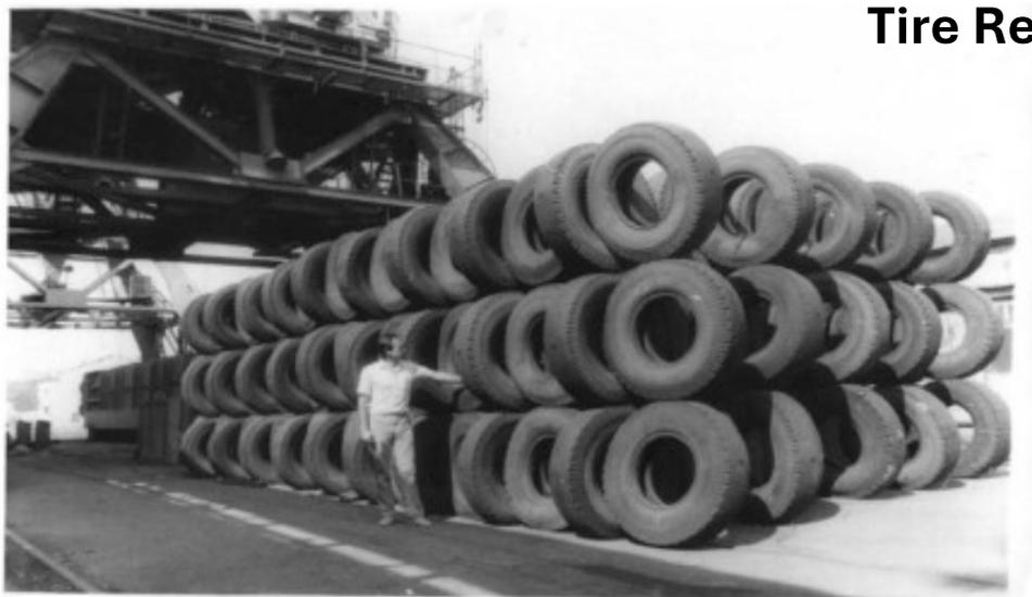
Figure 12.3 Tire reef prior to deployment in the Black Sea.
