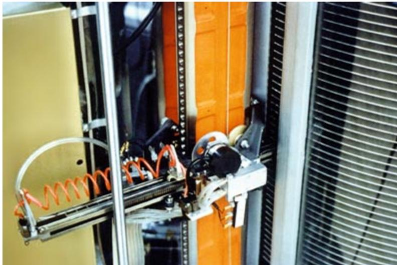
**Figure 1** First computer disk drive built by IBM in 1956 as part of RAMAC. On the right side of the image, some of the 50 platters are seen. In the center of the image is a pneumatically controlled access mechanism. [1]
